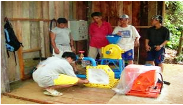
Fig. 8 Community-based hydro power installations in Sabah and Sarawak (SSS 2013)
