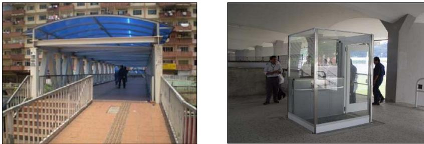
Fig. 2. (a) ramp into a bridge building; (b) an example of a quick solution – A platform lift in Taman Tasik Titiwangsa
