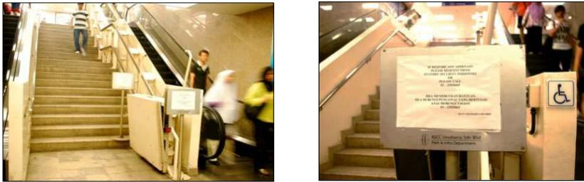
Fig. 5. (a) platform lift installed at the main staircase to the light railway transit station at a major transportation hub at KLCC (Source: Authors, 2011); (b) shows the instruction on a typed small piece of paper as the notice on how to use the platform lift, clearly lacking in contrast and font size to read for disabled persons (Source: Authors, 2011)
